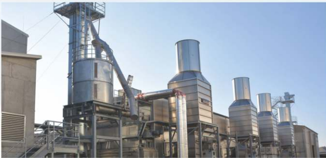
Biomass Power Plant at SAFE® Bedding (Germany)
